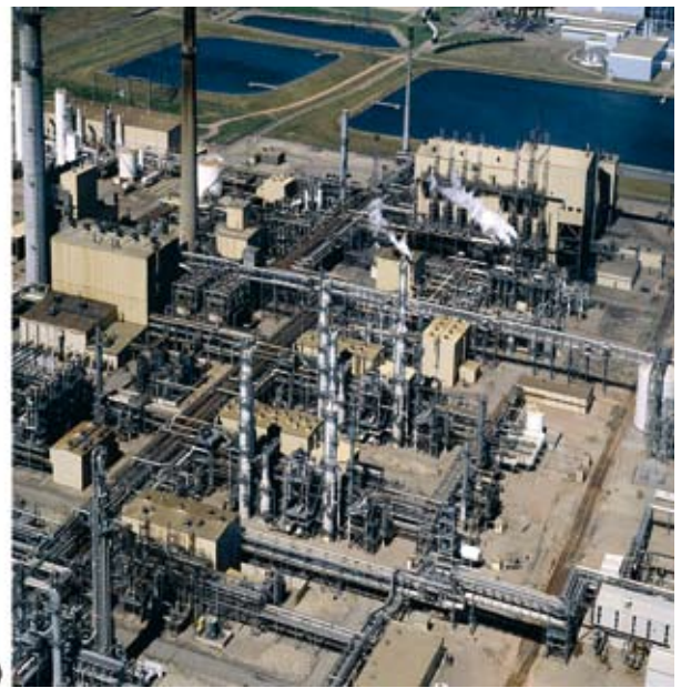
Figure TS.4. (a) CO 2 post-combustion capture at a plant in Malaysia. This plant employs a chemical absorption process to separate 0.2 MtCO 2 per year from the flue gas stream of a gas-fired power plant for urea production (Courtesy of Mitsubishi Heavy Industries). (b) CO 2 pre-combustion capture at a coal gasification plant in North Dakota, USA. This plant employs a physical solvent process to separate 3.3 MtCO 2 per year from a gas stream to produce synthetic natural gas. Part of the captured CO 2 is used for an EOR project in Canada.
